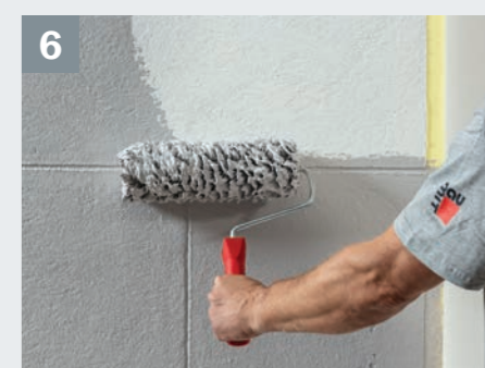
6 After the CreativTop Pearl has dried for at least 24 hours*, apply a single coat of Baumit StarColor (diluted 20% with water) in shade 0927 or 0447. Processing is either wet-on-wet across the field or seamlessly from joint to joint.
