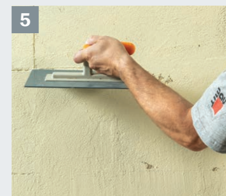
5 After stiffening, the joints are restructured again using a plastic float.
