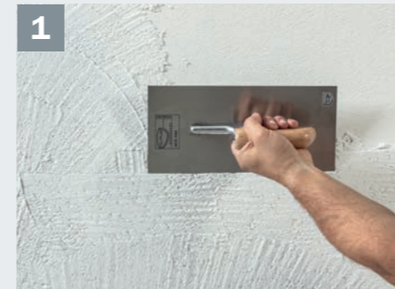
1 Baumit CreativTop Trend comes with a stainless steel trowel applied over the entire surface, coarsely rubbed....
