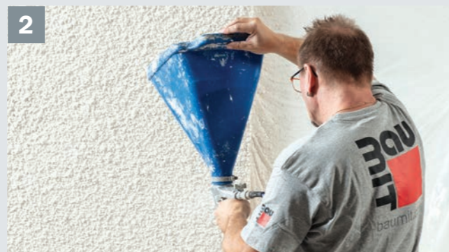
2 After 12 hours apply a second layer of CreativTop Max.
