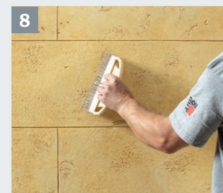
8 ...immediately wipe away with a glaze brush.
