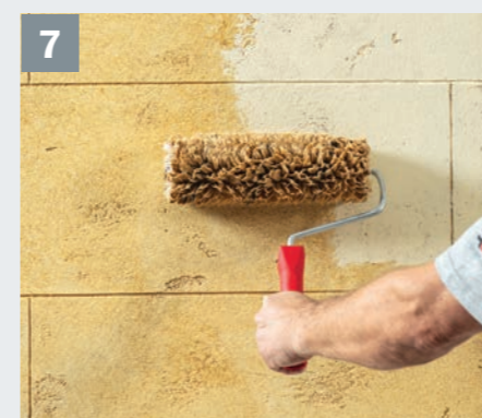
7 Apply Baumit Lasur in colour 735L...
