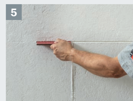
5 After hardening, the joints are reworked again with sandpaper so that in the finished appearance even joint dimension shows.
