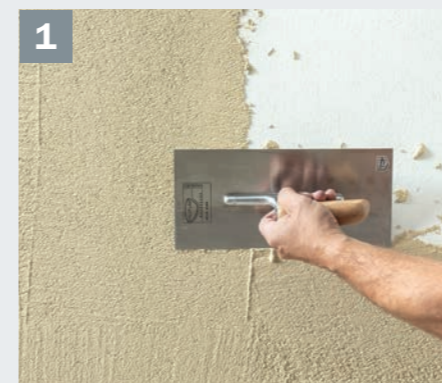
1 Baumit SilikonTop K 1.5 in colour 0185 is applied over the entire surface with a stainless steel trowel raised and rubbed...
