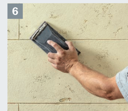
6 After standing for 24 hours* roughly sand the surface and the joints with 16-grit sandpaper.
