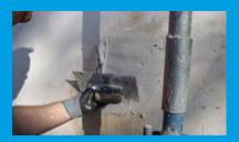
20 mm, with high salinity of 30 mm. The fresh restoration plaster is now pulled with a grape brush or a surface smoother and roughened with a cleaning comb. Danger! Protect the restoration plaster layer from drying out too quickly!
