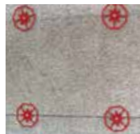
The Baumit adhesive anchors are offset in height, maximum 40 x 40 cm.
