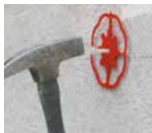
The Baumit adhesive anchors are inserted into the borehole and secured with plastic nails.
